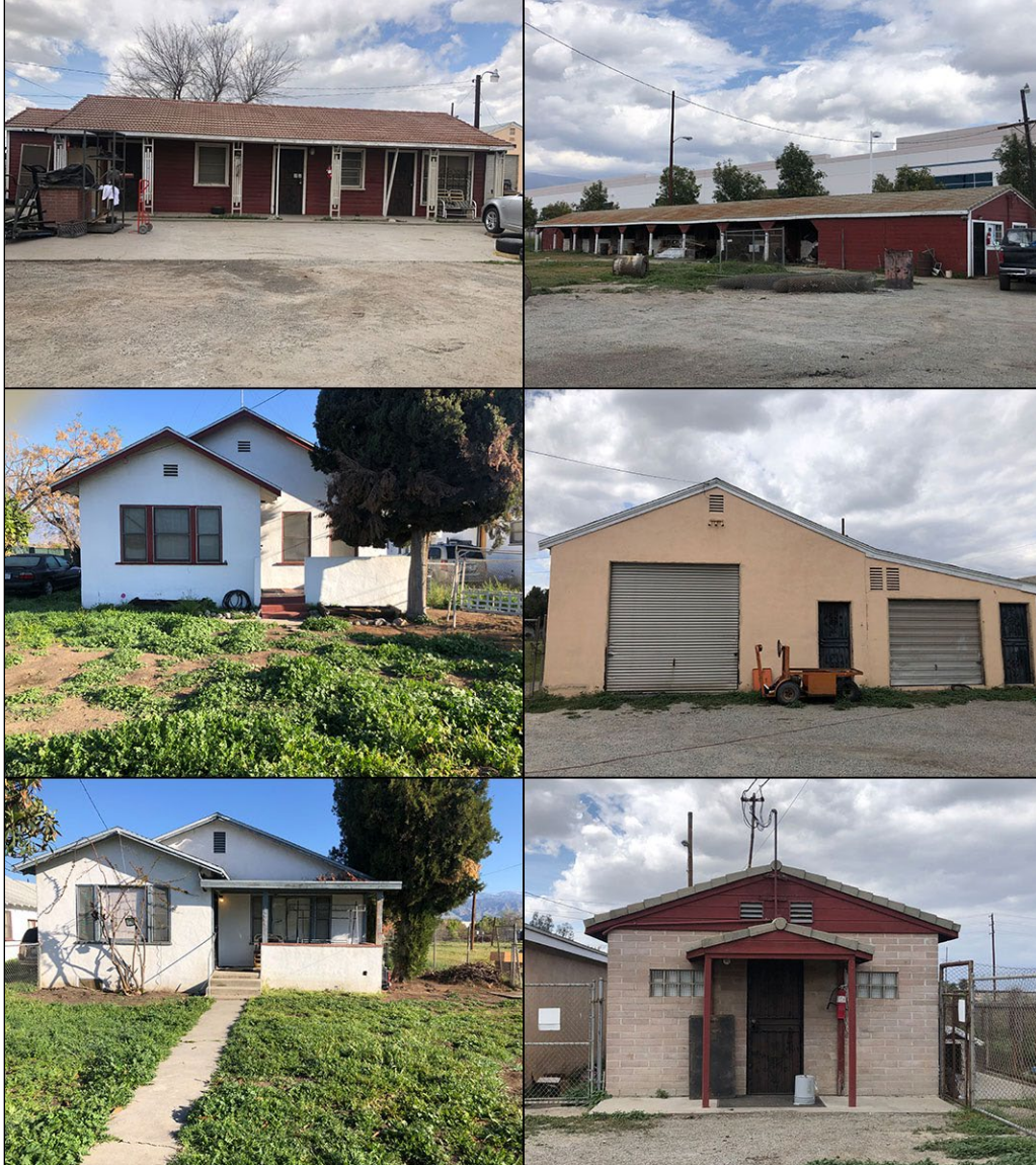
Buildings on the Bergman Ranch property. Clockwise from top left: the Ranch-style residence behind the original farmhouse (see photograph on p. 1), view to the west; stable, view to the northeast; workshop/garage, view to the west; modern brick shed, view to the north; the two nearly identical residences in the southwestern portion of the property, view to the north. (Photographs taken on March 16 and 25, 2021)
